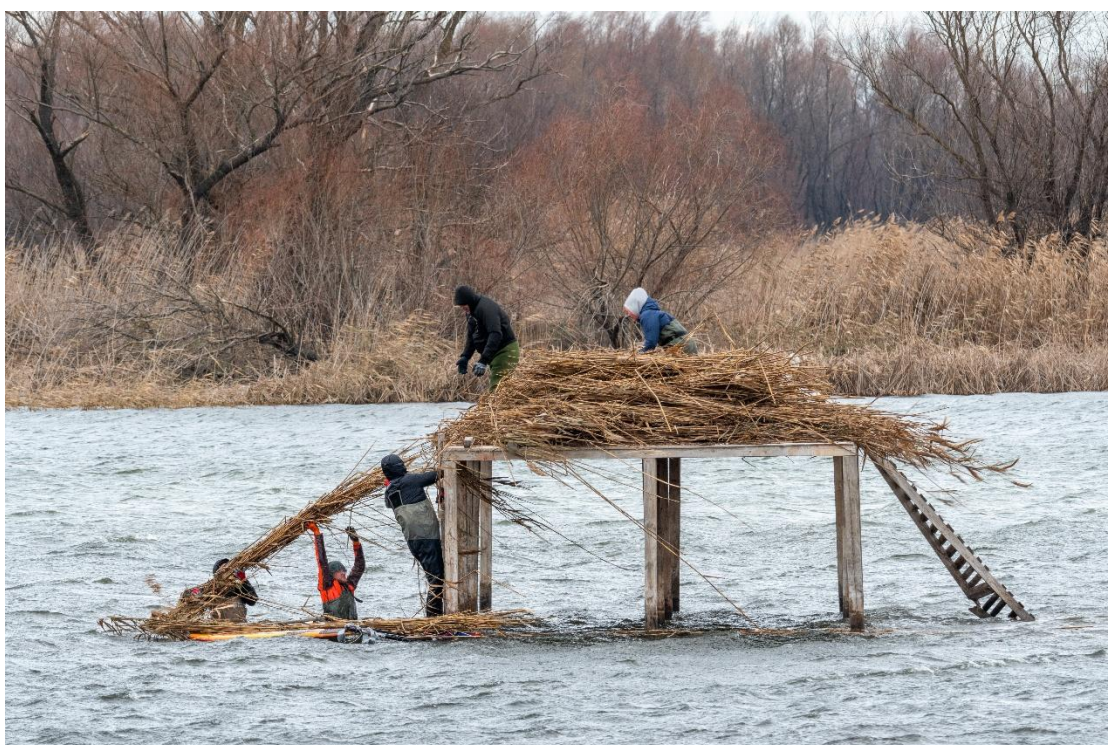
Maintenance and repair activities on the platforms during the winter months, photo credit: Damyan Petkov
