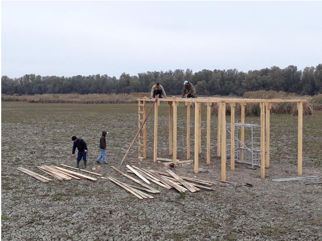
Construction the wooden platform at Peschina marsh (Persina Nature Park), photo credit: Svilen Cheshmedzhiev
